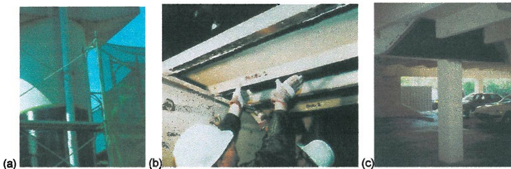
Figure 1 Composite overlay repair/upgrade of civil infrastructure: (a) circumferential reinforcement of a bridge column; (b) bending reinforcement of a concrete deck; (c) shear reinforcement of a parking deck beam ( Composites Design and Applications , Winter 1996 and January/February 1997).
